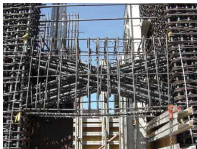
Fig. 1: Typical diagonally reinforced coupling beam (photo courtesy of Rémy Lequesne)
